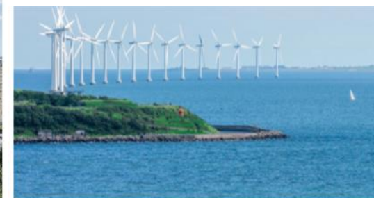
Middelgrunden offshore wind farm, 3.5 km from Copenhagen, Denmark. When built in 2000, it was the largest offshore wind farm in the world, at 40 MW. Wind generation will provide 50 per cent of Denmark's electricity by 2020. Such high shares of wind generation will be made possible, in part, by the country's extensive district heat networks.
