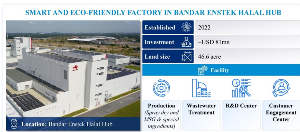
Figure 9: Factory in Bandar Enstek Halal Hub
