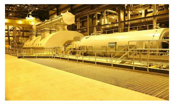
Figure 17 – Longview Turbine and Generator Set<sup>16</sup>
