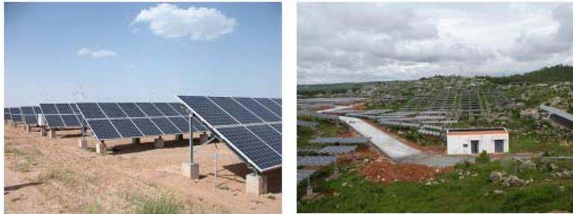
Fig. 3-4 Fixed PV matrix on flat ground and fixed PV matrix on the slopes
