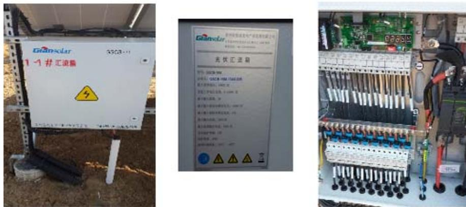
Fig. 5-4 Combiner box used in this project
