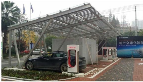
Fig. 1-14 Photovoltaic carports and charge piles
