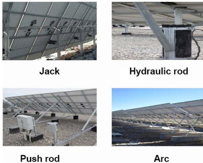
Fig. 2-8 Comparison of 4 adjustable fixed stands
