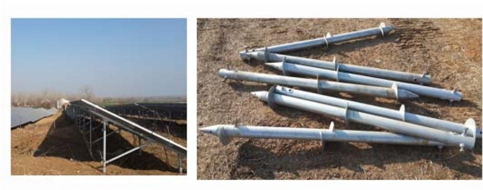
Fig. 5-6 Holder and foundation used in the 16MW project
