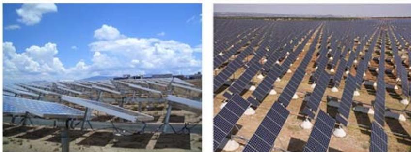
Fig. 3-9 Inclined homotaxial hour angle tracking matrix (W-E rotation)
