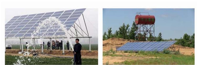
Fig. 1-20 Photovoltaic water pump
