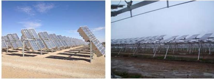
Fig. 3-10 Bi-axial tracking matrix (simultaneously tracking hour angle and declination angle)
