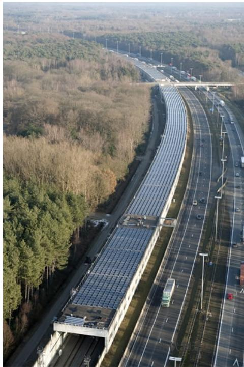
Fig. 1-11 PV railway tunnel
