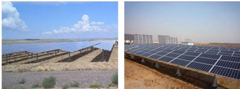
Fig. 3-8 Flat homotaxial hour angle tracking matrix (E-W rotation)
