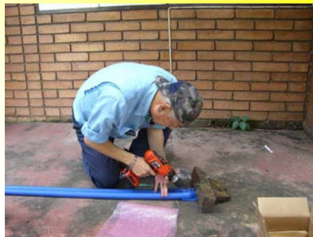
Putting temperature sensors inside/outside heat exchange tube (U-tube)
