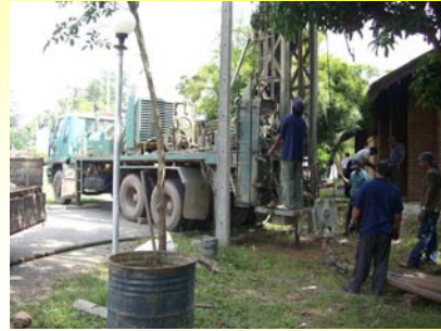
Drilling of heat exchange borehole, 2006.10.17
