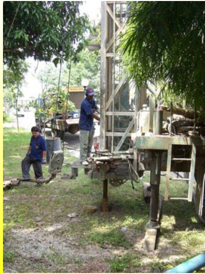
Drilling of heat exchange borehole, 2006.10.17
