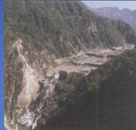
Shiraiwa sabo dam
