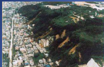
Immediately after a slope failure disaster
