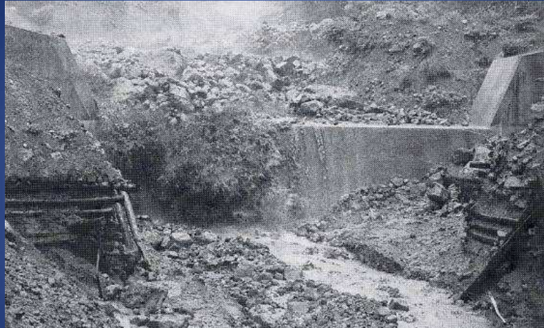
Kamikamihorisawa, Yakedake Volcano on August 3, 1976 (width of waterway of groundsill: 16 m; tip speed: 3.8 m/sec)
