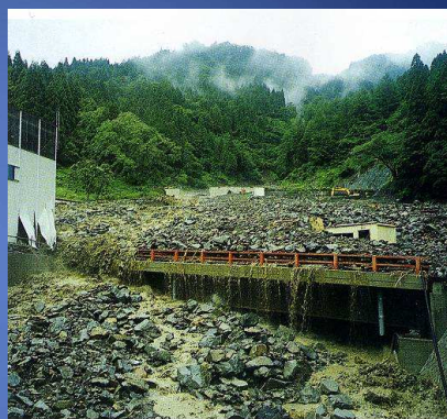
After the occurrence of a debris flow on the morning on July 12, 1995
