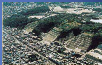
Immediately after the completion of the works
