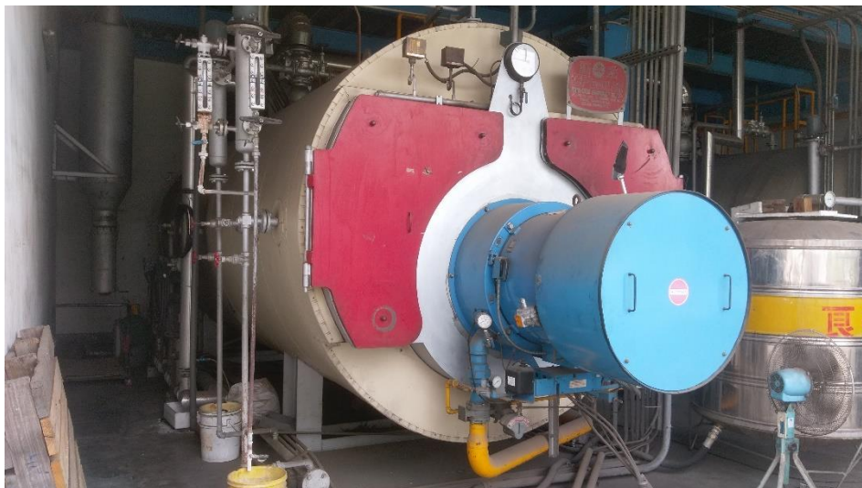
Figure 2.25 Packaged boiler fired with natural gas
