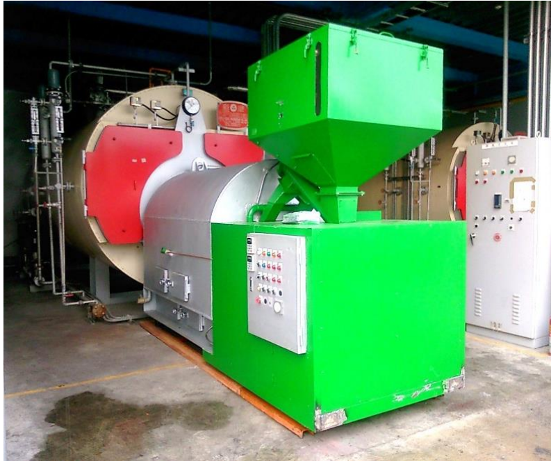
Figure 2.28 Bio-pellet steam packaged boiler
