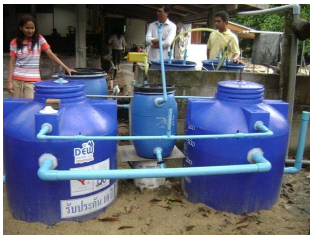
Figure 4. Biogas Innovation from Rubber Sheet Wastewater in Pattalung Province, Thailand
