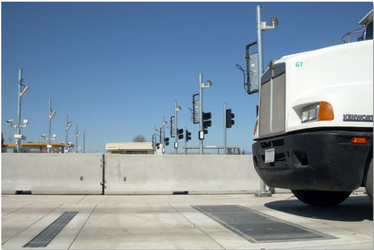
Figure 13: Typical WIM set using in ground bending plates to record mass
