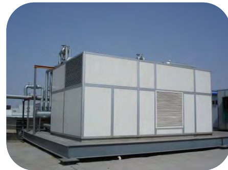
Figure 2 evaporative cooling and mechanical refrigeration compound high-temperature chiller
