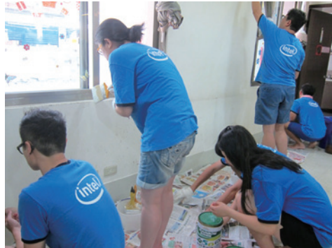
Re-painting the walls of a Shelter for the homeless.
