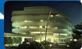
Passive House Technology Experience center 15022m 2
