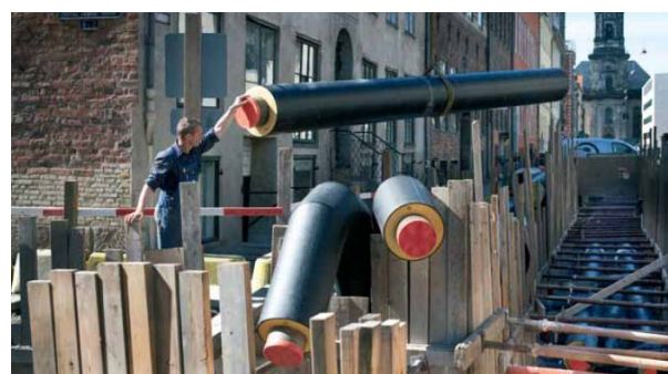
Figure 7.2.2 Thermal Insulation of High-temperature Heating Pipe Network
