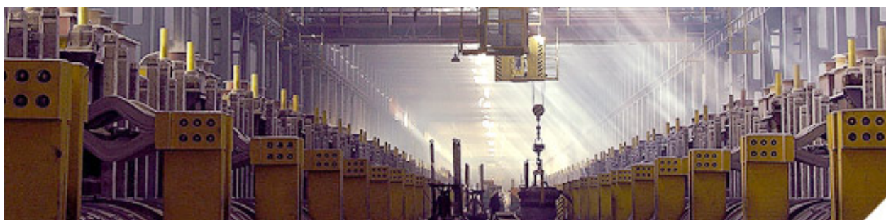
Figure 16.1.2 KrAS (Krasnoyarsk Aluminum Smelter) Factory
