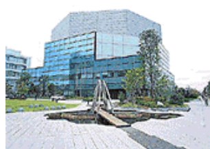
District heating and cooling plant
