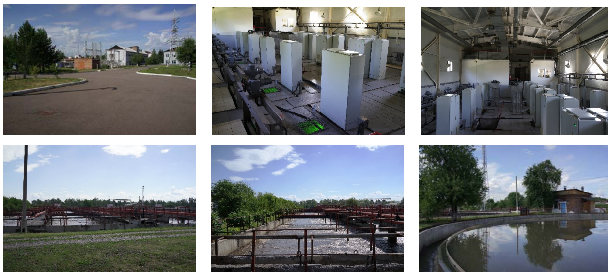
Fig 12.1.1 Sewage treatment facility in Krasnoyarsk (Bacterial treatment facility)
