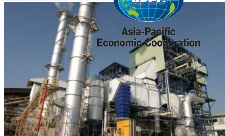
Bagasse Fired Cogeneration (on-grid 29MW) – Phu Khieo Bio-Energy Co. Ltd. Thailand Photo courtesy by COGEN 3 Info Sheet
