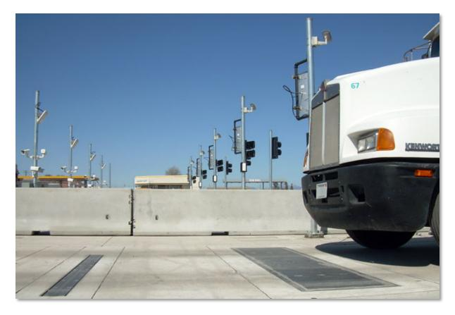
Figure 13: Typical WIM set using in ground bending plates to record mass SOURCE: http://www.irdinc.com/pages/its-solutions.html
