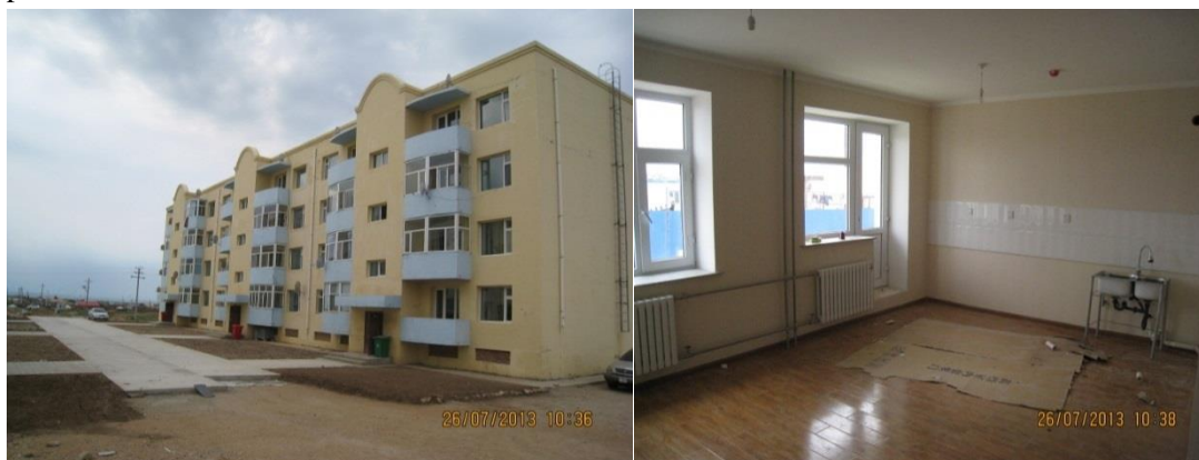
Figure 3-14 Clean and commodious family dormitory buildings; there are heating installation, tiles, solid wood floor and others.
