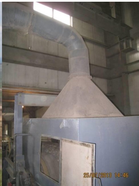
Figure 3-9 Dust absorption facility in ore-breaking workshop
