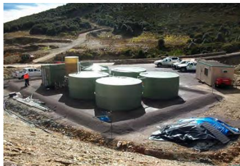
Figure 5-8 Drinking water treatment plant in South Hercules
