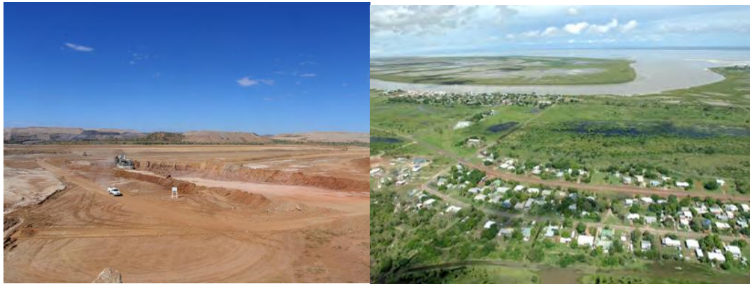
Figure 5-1 The No. 10 sediment dam of the Century mine lot
