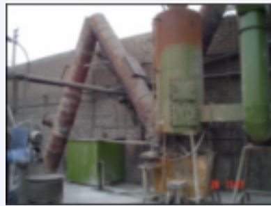
Auxiliary tank for decantation
